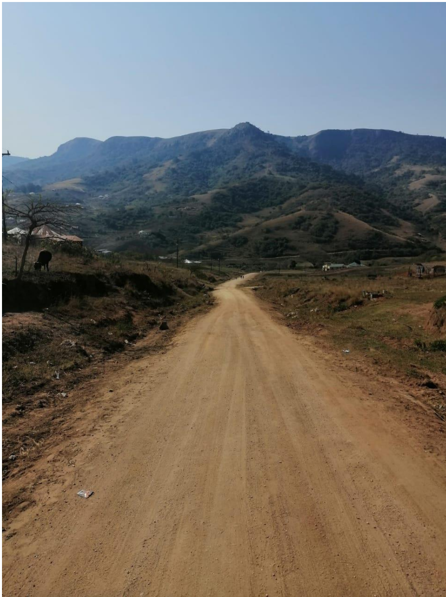
Road conditions on D1006
