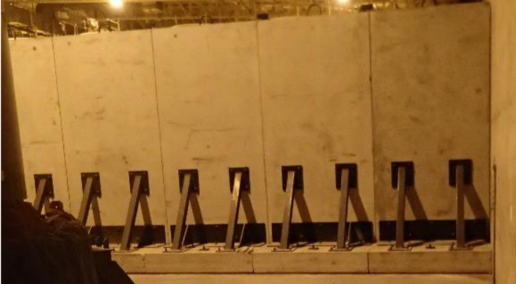
Figure 5: Pre - Cast Concrete Shield Panels at Low Level Waste
