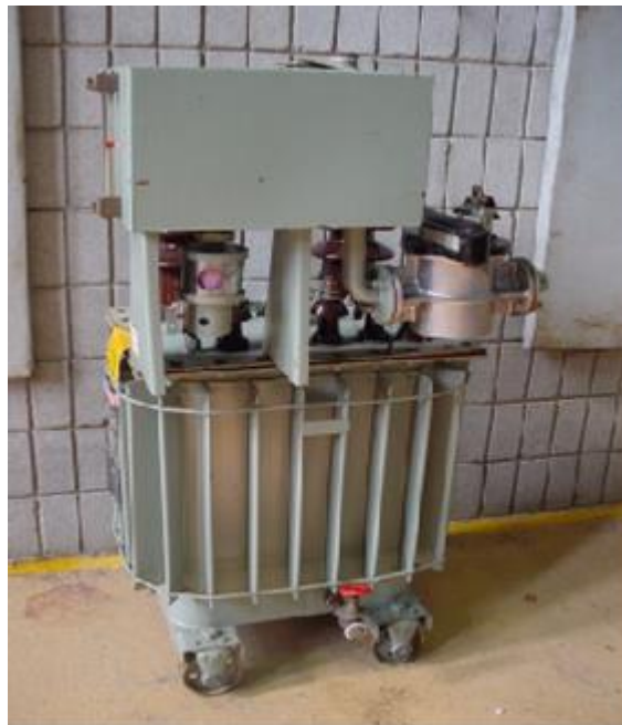
Figure 1: Existing Single Phase Excitation Transformer, (3 per unit)
