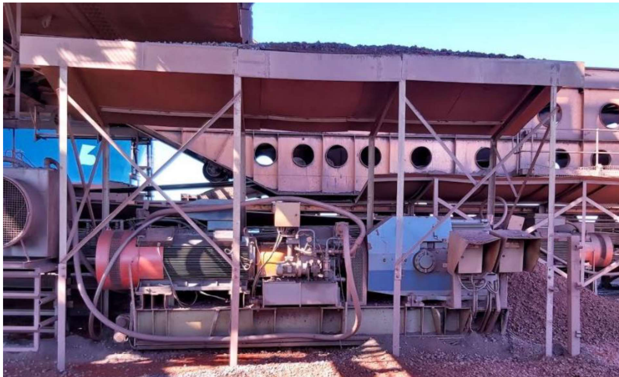
Figure3: Different Views of Existing Drive Canopy
