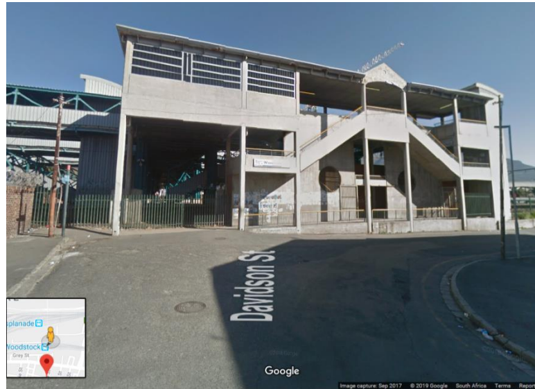
Figure 2: Street Entrance to Woodstock Station on Harbour Side
